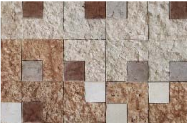
Figure 7: Detail of the external revetment of the sacellum in the Castelvecchio Museum, Verona (source: [11])
