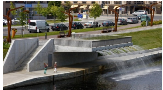
Fig. 35 The Driksa River promenade in Jelgava [https://www.redzet.lv/images/large/7/44/V-889-14.jpg]
