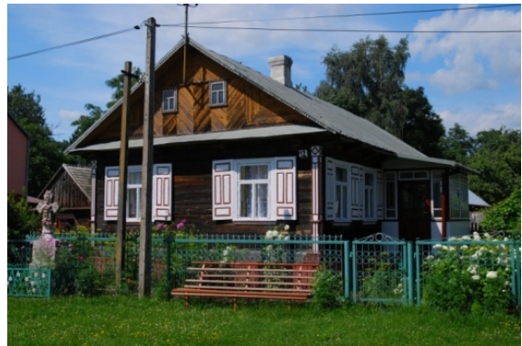
Fig. 4 Traditional house in Podlasie in Poland - the archetype of architectural form in search of expression of new forms of residential architecture in a given place
