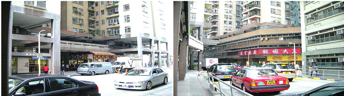
Figure 8: Shops on ground and residence on floors above
