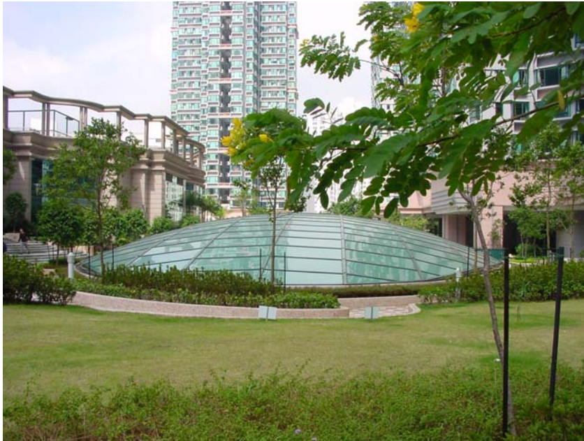
Figure 13: Green space on podium
