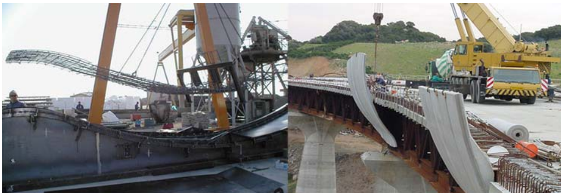
Figure 6: Construction and assembly of the sinusoidal concrete shields on site
