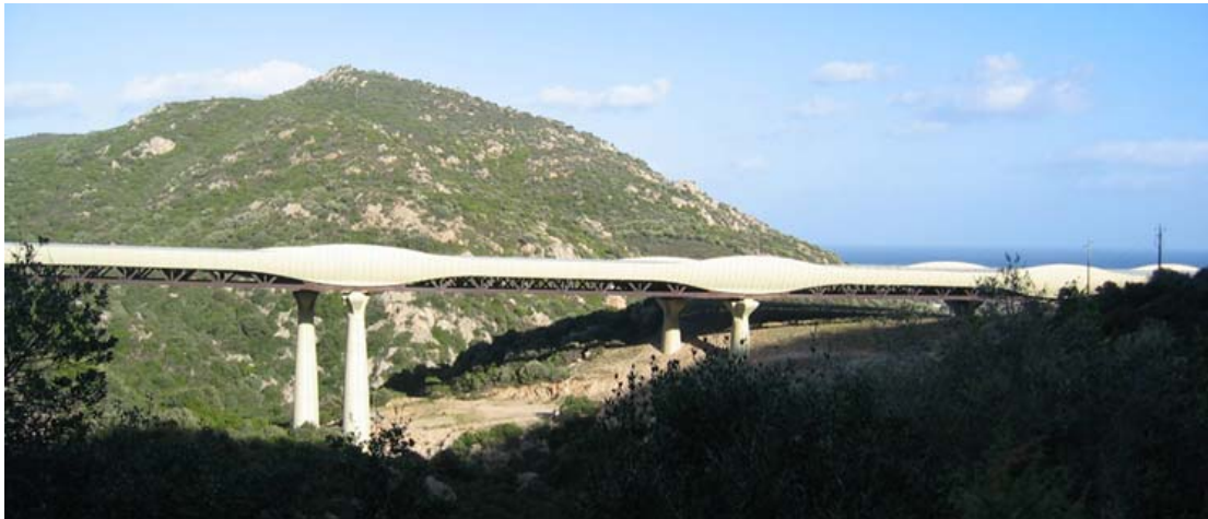
Figure 2: View of the Li Cuponeddi viaduct
