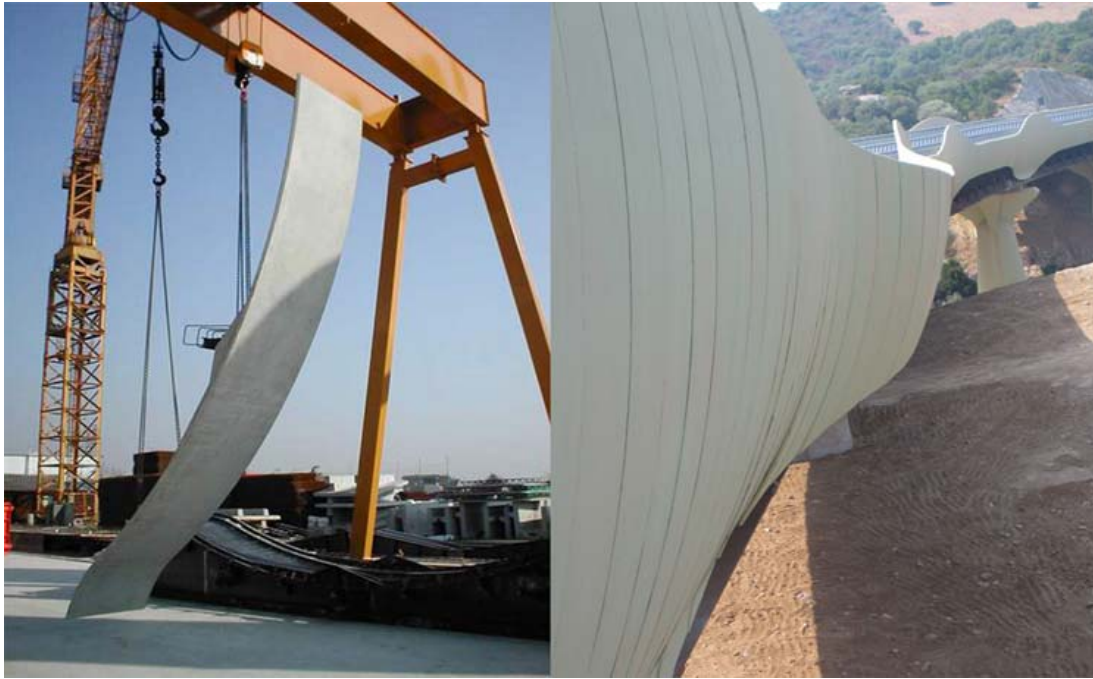
Figure 7: View of one concrete shield component and the overall sinusoidal enveloping shape
